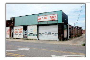
replacement of the storefront and the addition of metal siding to the upper facade
